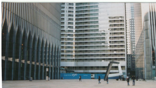
Figure 2. WTC site before construction of the Memorial , looking west. Tower One is on the right. Tower Two, on the left. Photo: E. Zimmerman.
